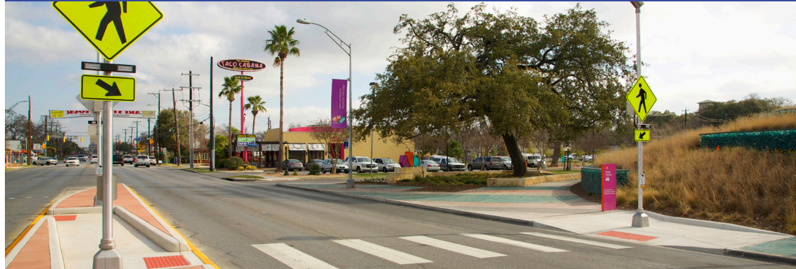
Recently installed Z-crossing on Broadway in front of the DoSeum Children's Museum
